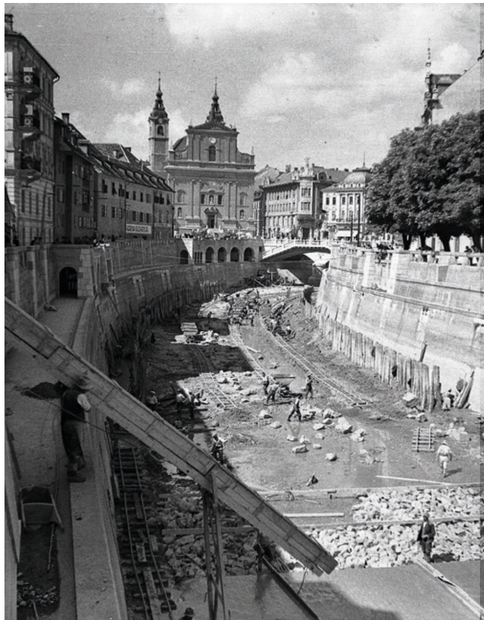
42. Regulacija reke Ljubljanice je po obsegu del pomenila večja gradbena dela v času gradbene krize v Ljubljani v začetku tridesetih let 20. stoletja. • According to the scope of works, the regulation of the Ljubljanica river represented major construction works during the construction crisis in Ljubljana in the early 1930s
